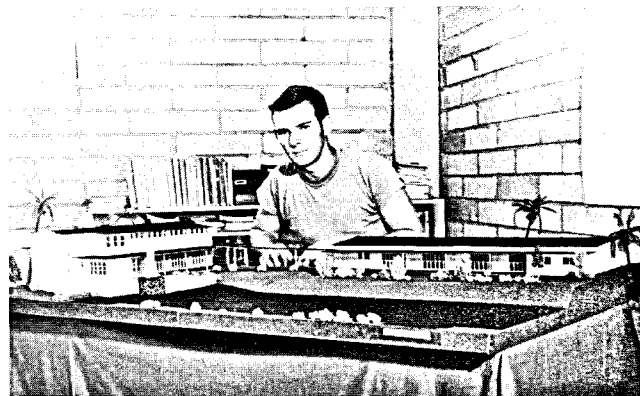
Roger (Sam) Manke, 17 years of age, and the son of Mr. and Mrs. Karl Manke, St. Stephen's Church, Wahiawa, made the scale model shown in the above picture, for the ground breaking service on December 22nd for the new parish hall that is to be built for the Church. It took him six weeks to complete the project, which was designed by the Vicar, the Reverend Howard B. Kishpaugh, and has a nursery, kitchen, 11 classrooms, a social hall and long lanai. St. Stephen's Church is shown at the left of the picture. So excellent was this model that he was asked by the head of the planned improvement area near the shopping center of Wahiawa, to make a more intricate scale model for this proposed area.
