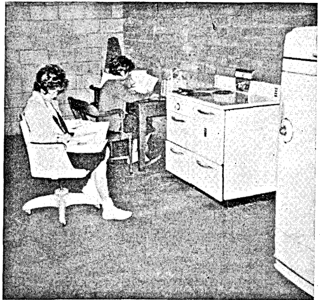
The Diocesan Warehouse proved a quiet spot for St. Andrew's Priory students to study for examinations before it was filled with articles for storage.
