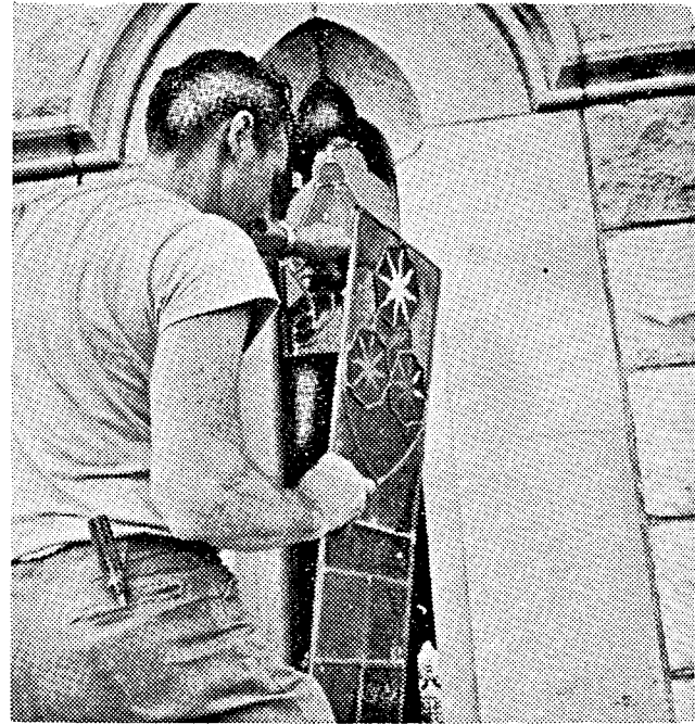
He holds upper section in place, slides in lower.
