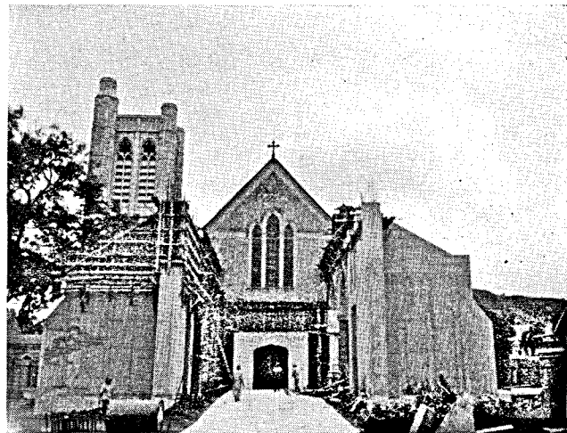
Looking into the Cathedral between the extension framework.
