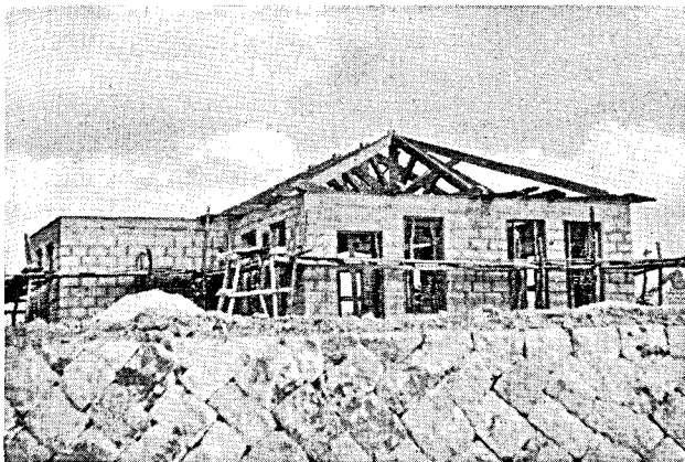
Rectory nearing completion on our Church property, Okinawa.
