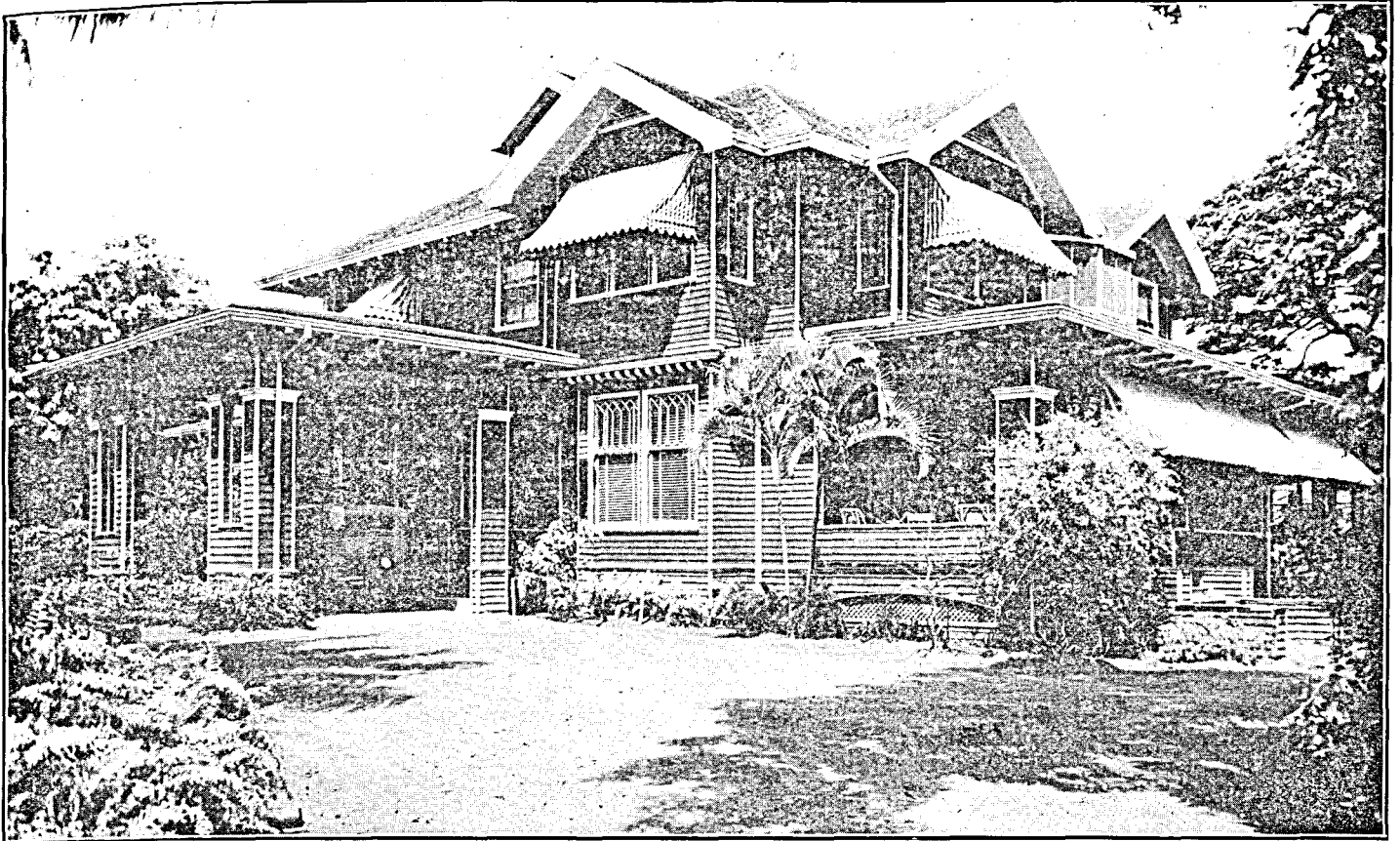
FACULTY RESIDENCE AND SCHOOL DINING HALL. FROM THE BROAD LANAI OF THIS FINE OLD RESIDENCE ONE GETS A MAGNIFICENT VIEW OF THE OCEAN
